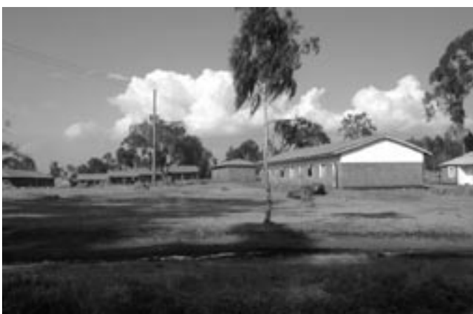
New classrooms at Murgwanza primary school, built as a direct result of debt relief
